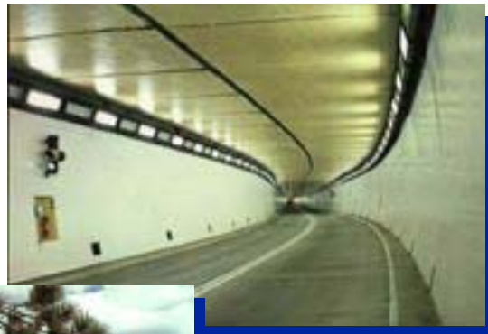
Tunnels and Bridges
